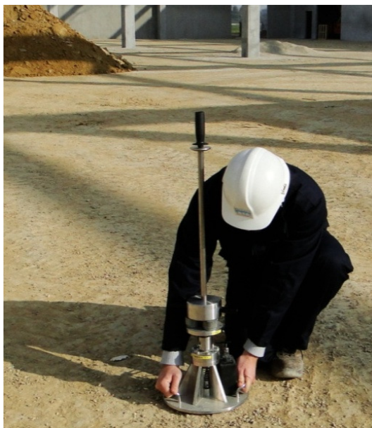
Figure 13 : Moving the plate to make good contact.
