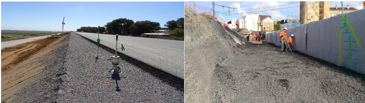
Backfill control by layer
